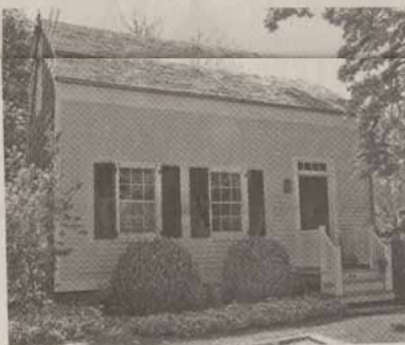
45 Glover Street (.1 acre) Single-family, 2-story residence
